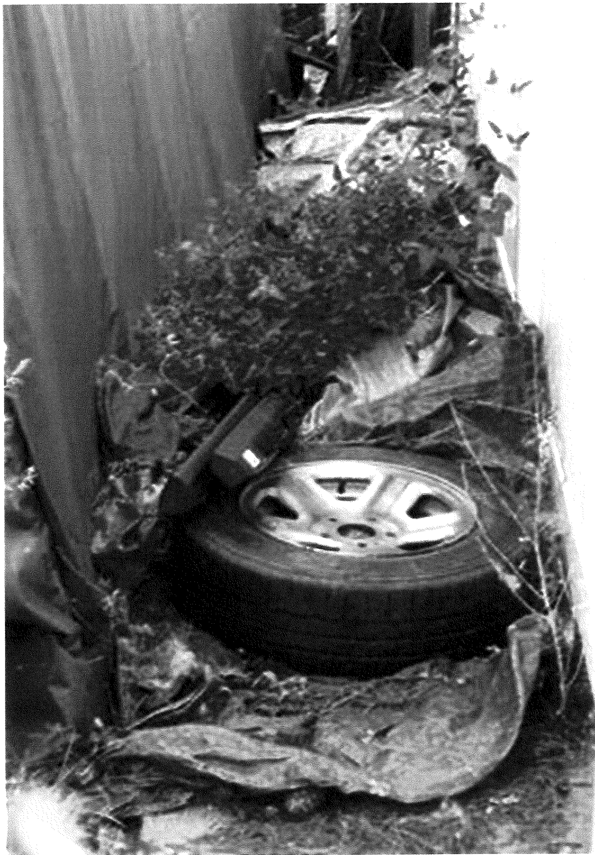
Glendale Gardens Bldg. 1308 Patio Walls w/ Dealership Trash 09.27.22
